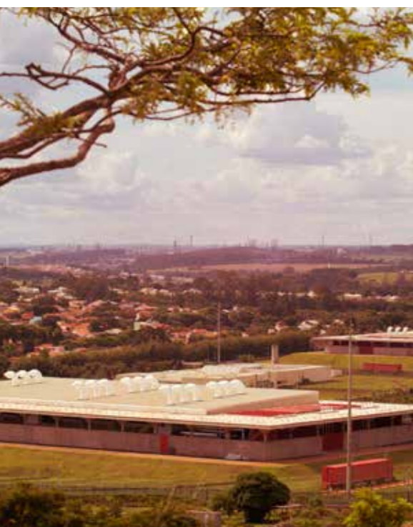
The new Santander Data Center in Campinas (SP)
